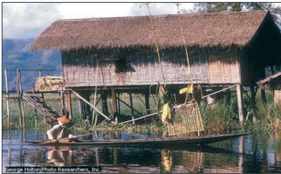
Use of stilts for raised floor above flood level
